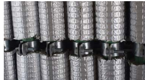
2 cm thermal polyolefin pipe insulation
