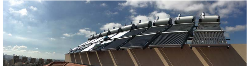
Solar water heating system
