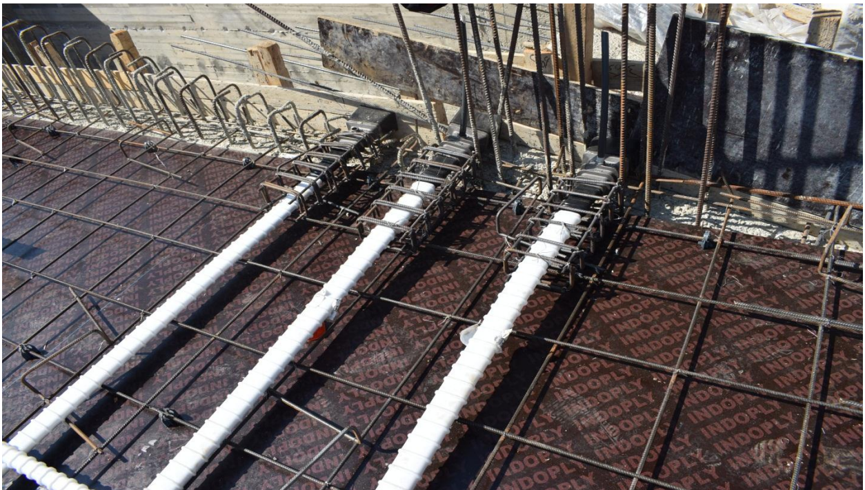
Enlarged View of the Pocket Forms of the XeD PT System with XF-20 Deviation Cone, XF-10 Anchor Head and PVC Black Tape
