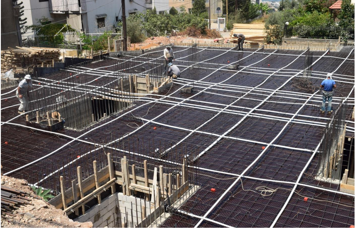
Upper View of the Basement 1 XeD PT Slab with anti-corrosive ducts
