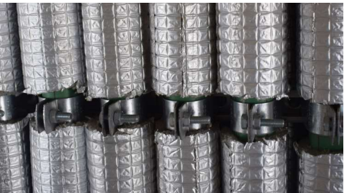
2 cm thermal polyolefin pipe insulation
